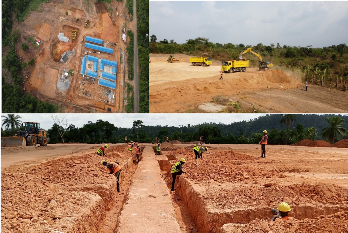
Figure 1: Ongoing construction activities at Segilola. (Source: https://www.thorexpl.com/ ).
